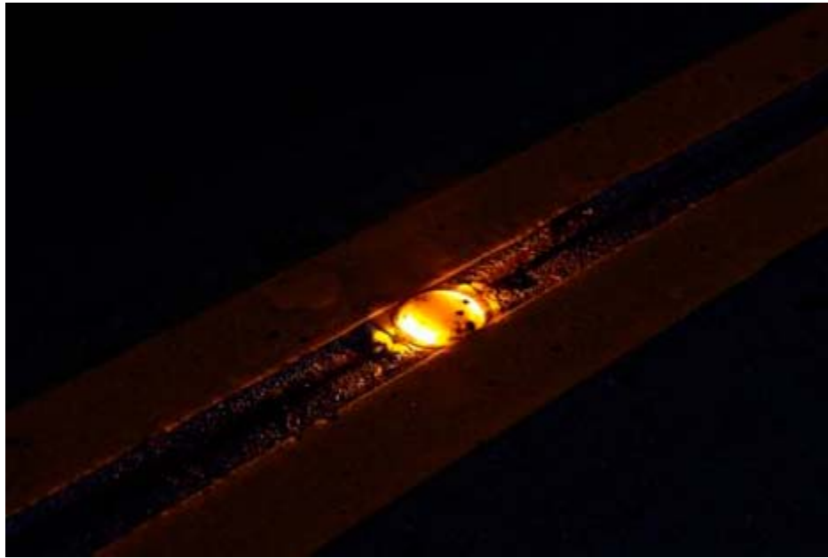
LED markers are lighted through inductive power transfer between the cable, which is fully sealed in the road surface, and a receiver circuit in the marker.
