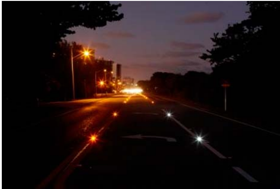
Overhead lighting, also part of the roadway's rehabilitation, is only turned on during the months when no sea turtle nesting occurs.
