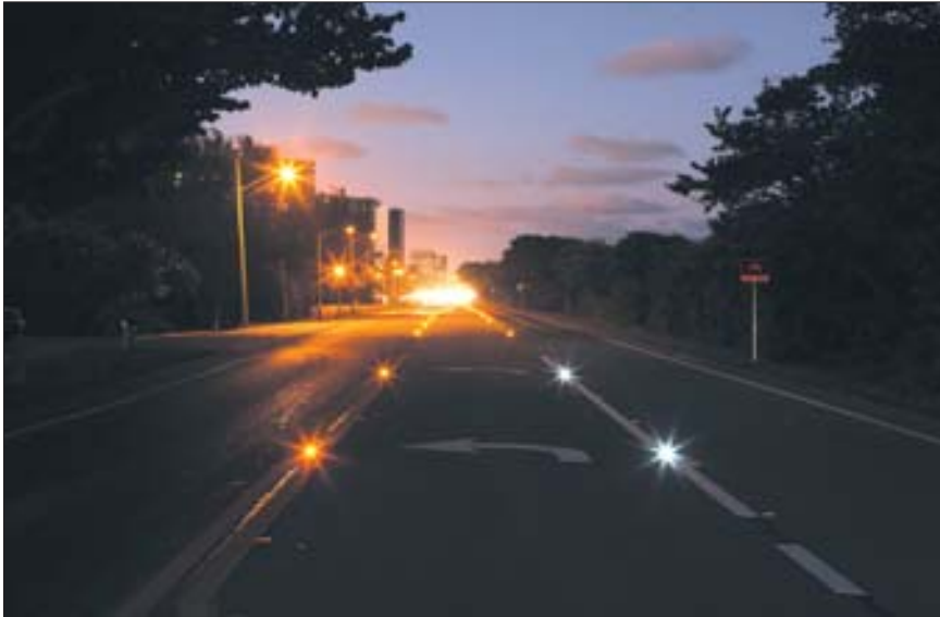
Only turned on during the months when no sea turtle nesting occurs, overhead lighting was also part of the roadway rehabilitation.
